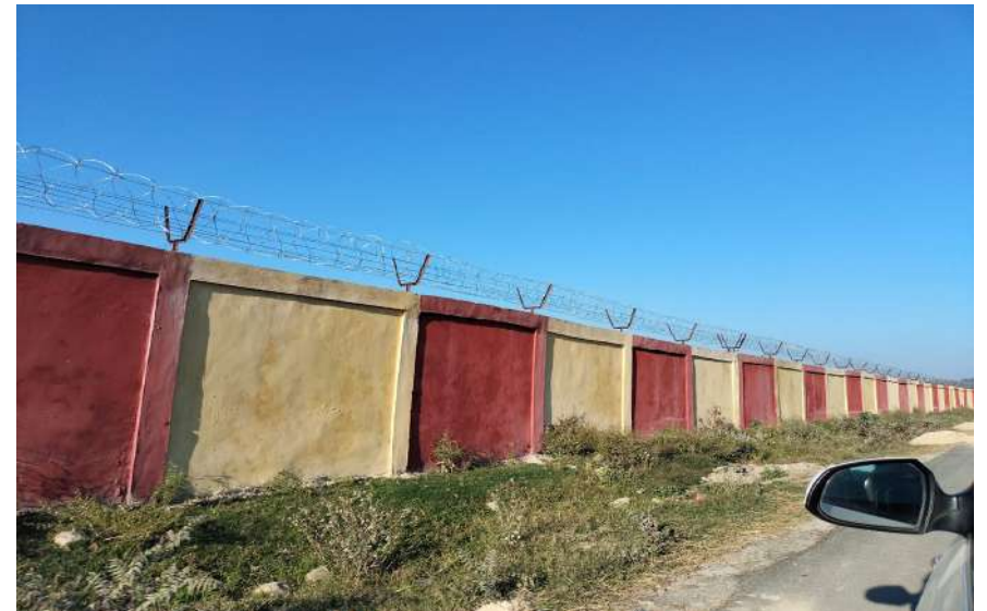
Pic: Donyi -Polo airport boundary wall- Arunachal Pradesh
